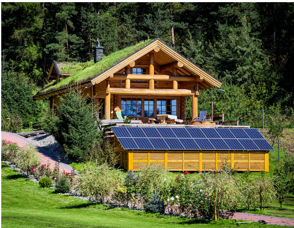
Home equipped with a photovoltaic (PV) system converting sunlight into electricity.
