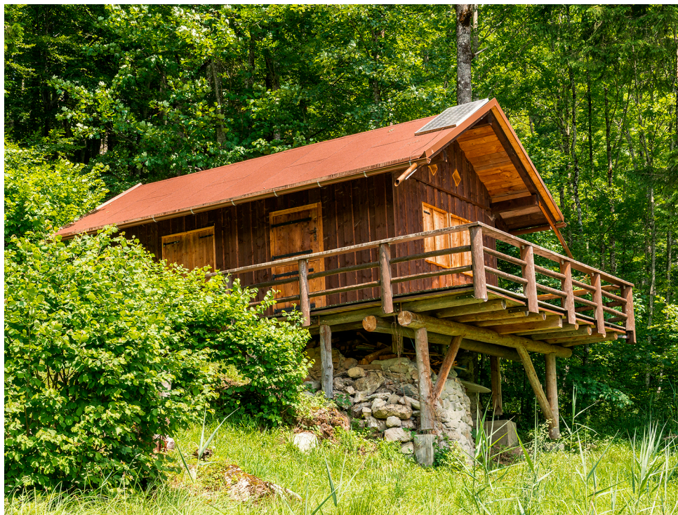
Figure 18. Small cabin powered by a stand-alone PV system.
